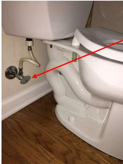
If you have an emergency with a leaking toilet, turn off the water supply quickly. Look for the water tube coming off the bottom of the tank and turn the knob to the right.
